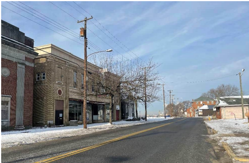
Vacant commercial storefronts fronting W Main St by the waterfront area.
