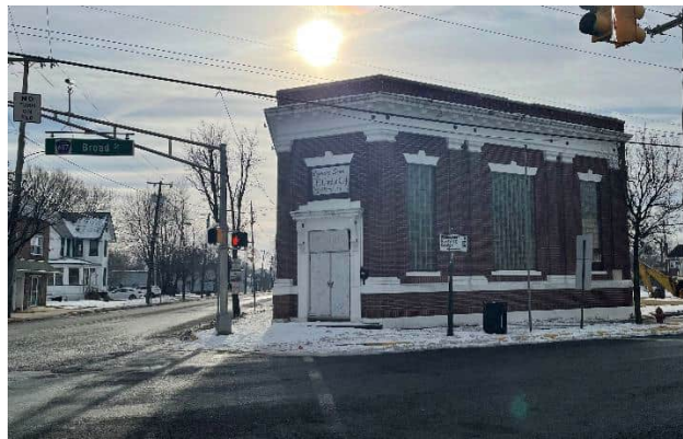
Vacant commercial storefront at the corner of Main St.-Broad St. intersection.
