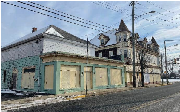
Vacant commercial buildings near the West Main St. & Broad St. intersection.
