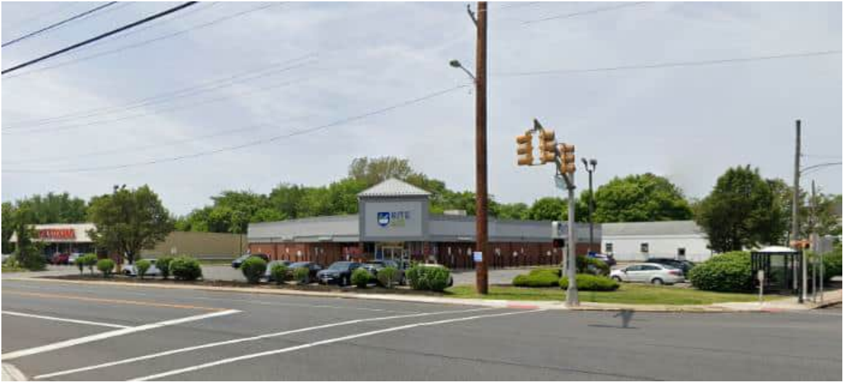
Intersection of Main St. and Route 130.
