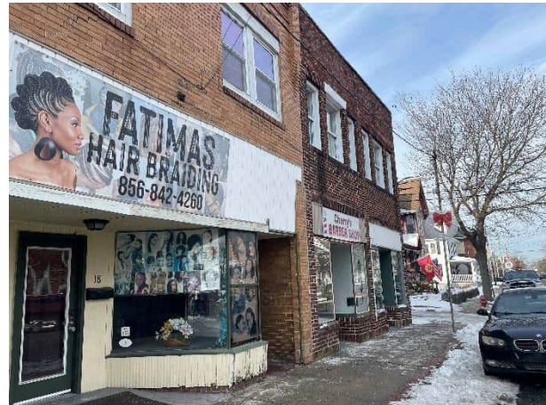
Existing storefront on W Main St.
