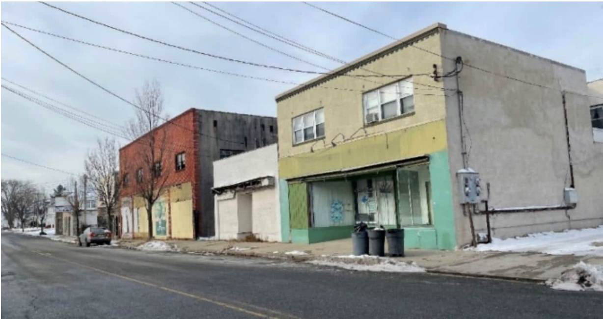
Vacant commercial buildings on Broad St. corridor.
